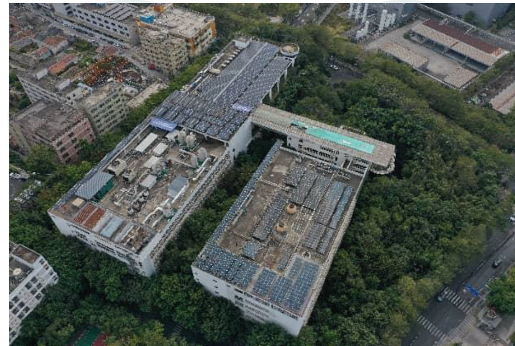
Rooftop photovoltaic installation (0.62 MW)
